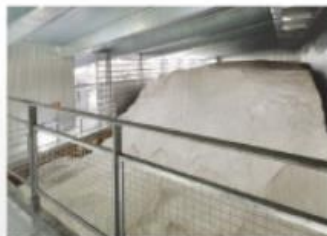
Hakkaisan Yukimuro that stores 1000 tons of snow
